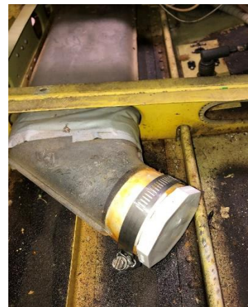
(right) Plug installed on aft heat plenum aft of the outlet for seats 3 and 4
