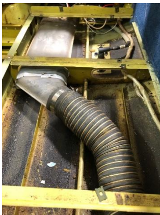
(left) Original duct
