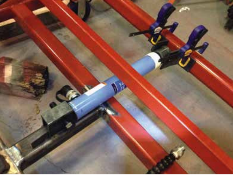
Tacking the fittings for the hydraulic ram.
