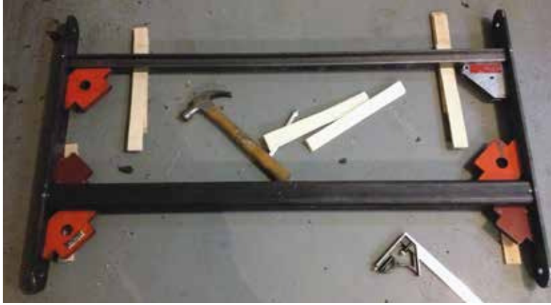
The lifting arm being fitted and tack welded.
