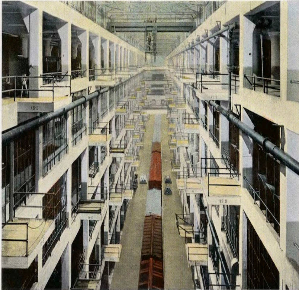
CRANEWAY IN NEW 6-STORY BUILDING, SHOWING LOADING PLATFORMS.
