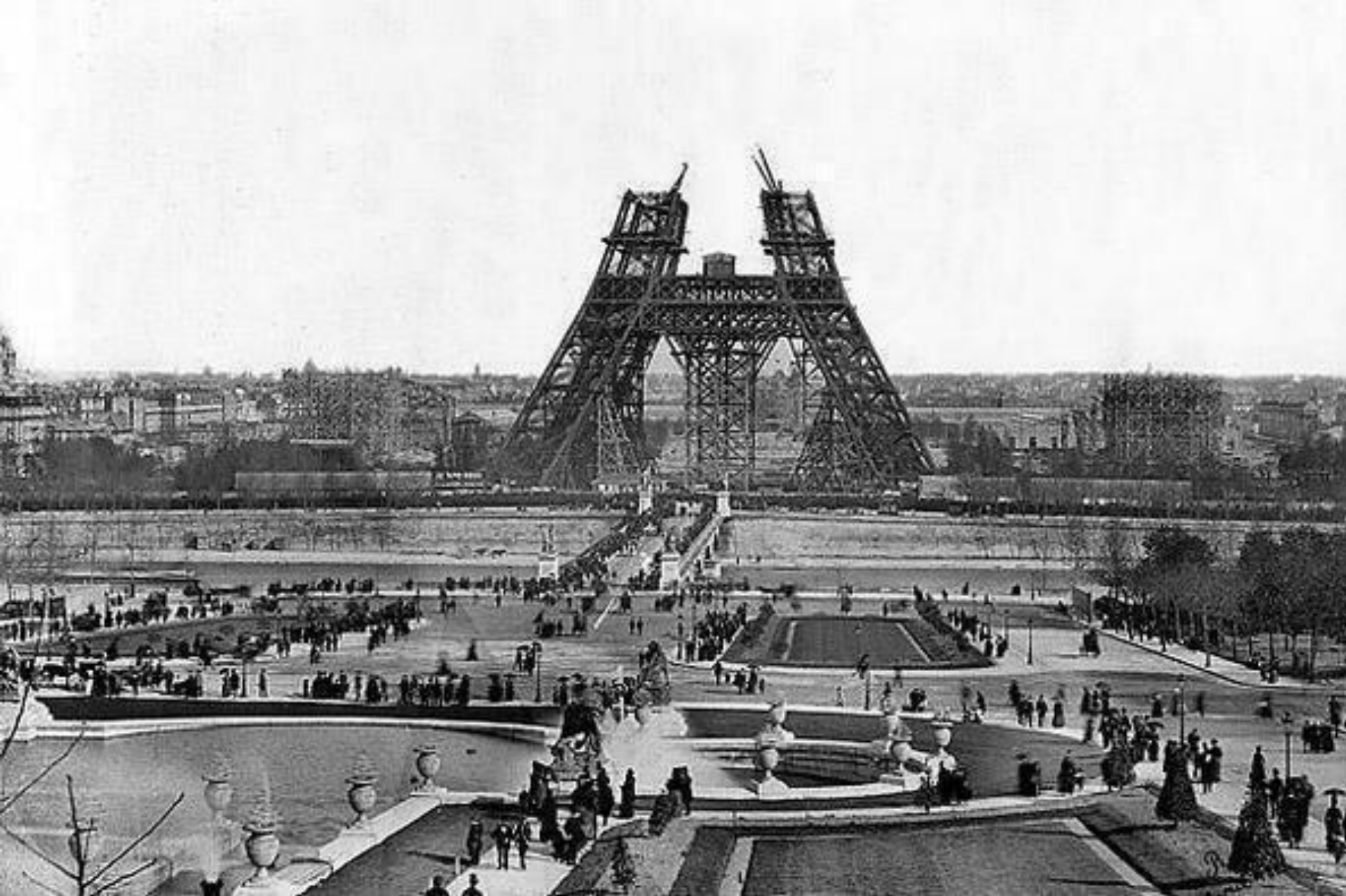
Construction of Eiffel Tower (1880)
