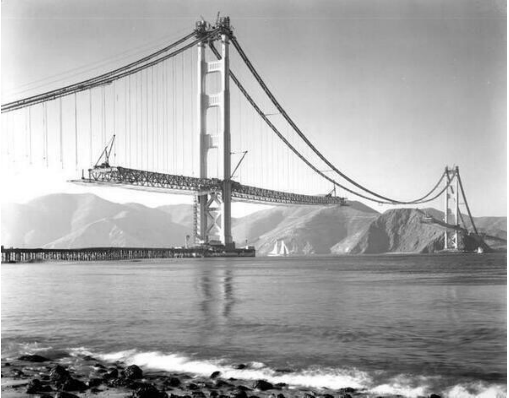
Golden Gate bridge construction, 1937
